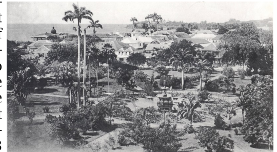
Arial View of the Square
