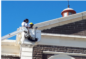
Structural engineer Danielle Steele is hoisted up to the building's parapet in the bucket of a SKELEC service truck
