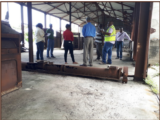
Trust officials visit the Spooner's site along with contractors and a Quantity Surveyor
